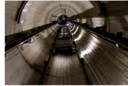
The distance between the 2 landings, traveled by elevator, is 31 meters through a shaft whose construction managed to keep together the new components with the old areas built from sandstone dated from the 18th century. The panoramic cabin of the STONE elevator has a round shape and is equipped with automatic glass doors with lower / upper stainless steel frame.
